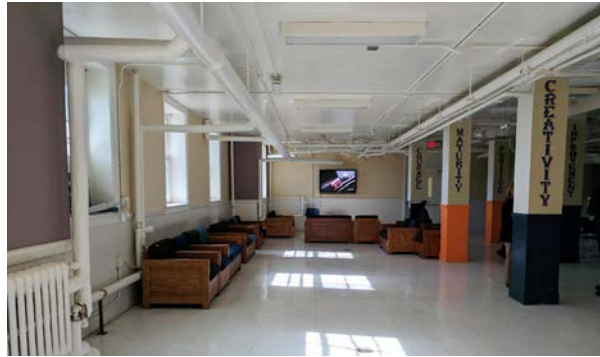
Existing Basement in Williams Hall
