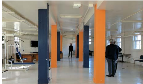
Existing Basement in Williams Hall
