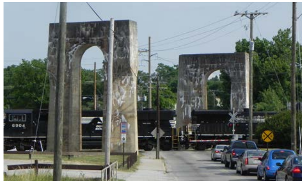
Existing View of Railroad Intersection
