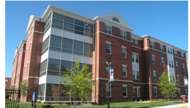
Existing Photo of Quad 1 Residence Hall
